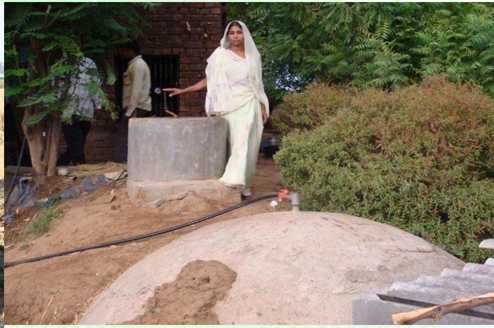
Sintex make Pre-fabricated HDPE material based 2m 3 Deenbandhu Model Biogas Plant
