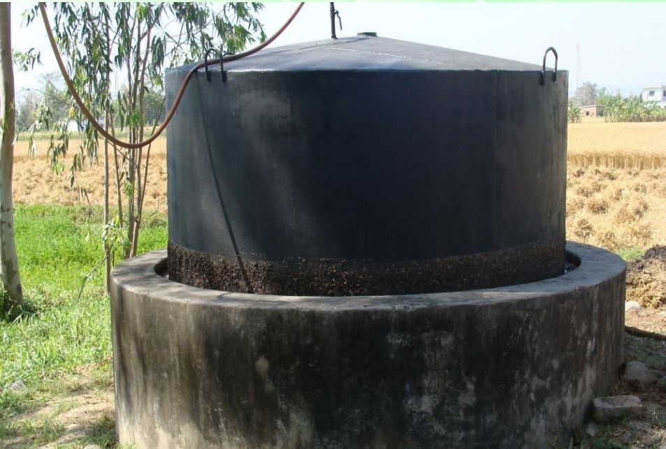
A Pre-fabricated RCC based Krishna model fixed dome Biogas Plant
