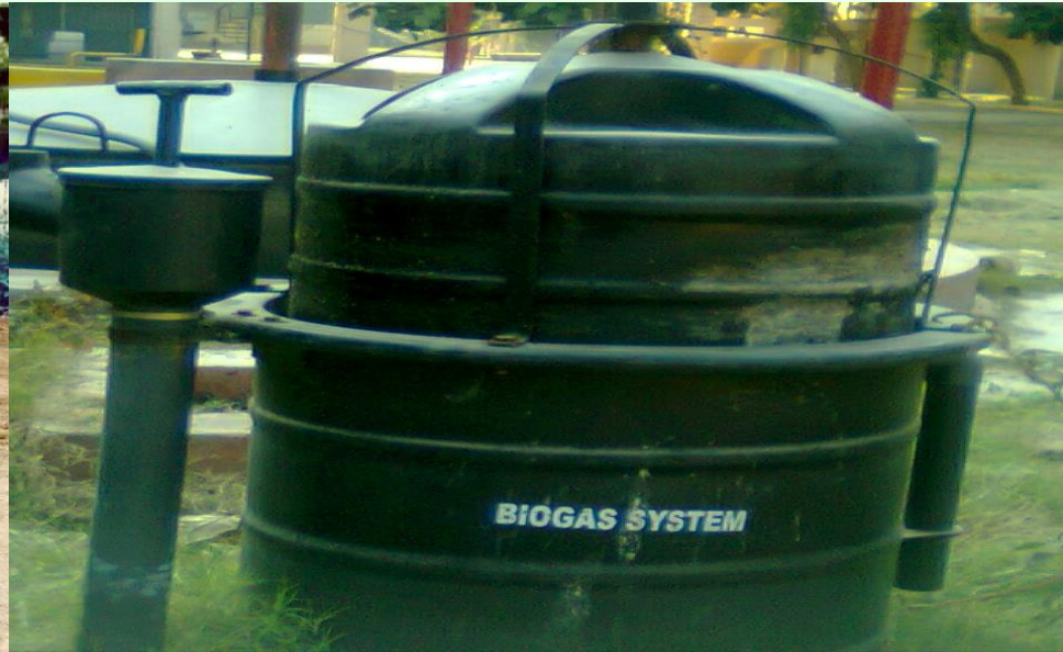
Sintex make Pre-fabricated HDPE material based 2m 3 Deenbandhu Model Biogas Plant
