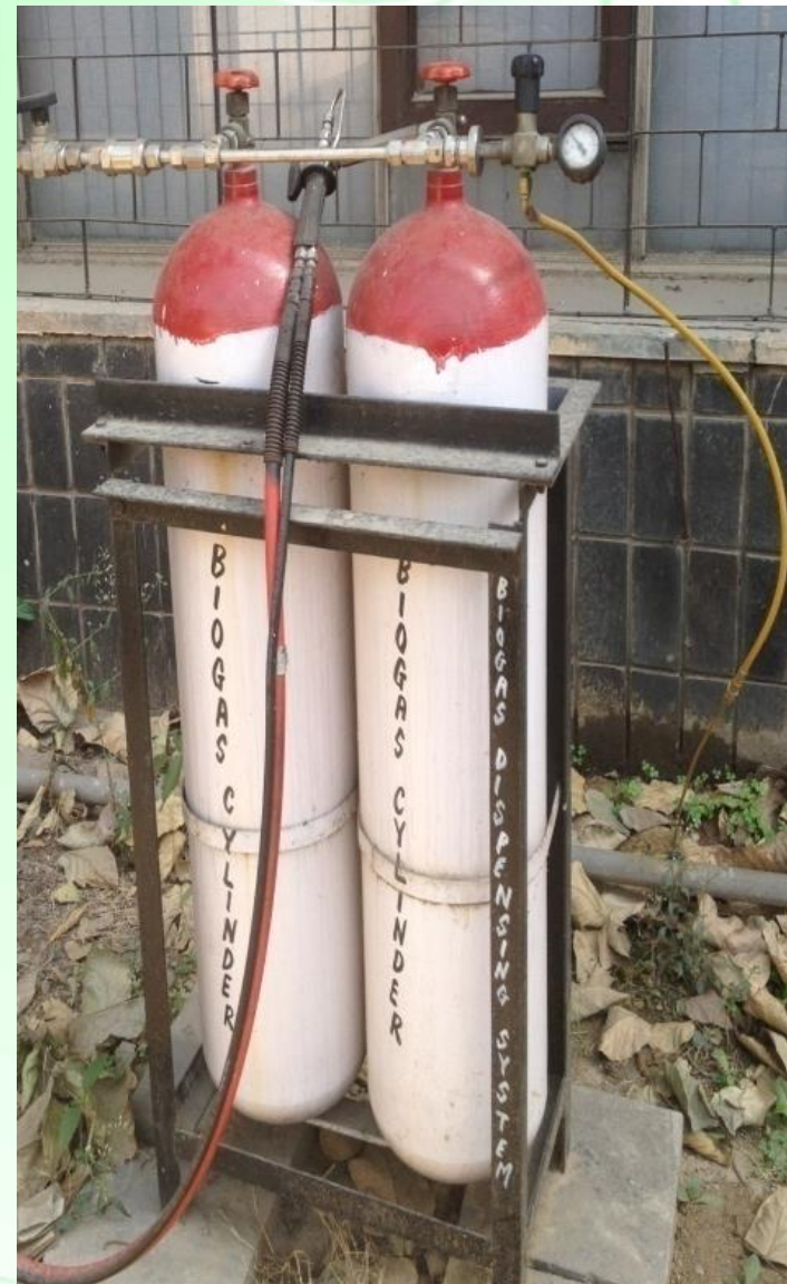
Two cylinder cascade for bottling of upgraded biogas
