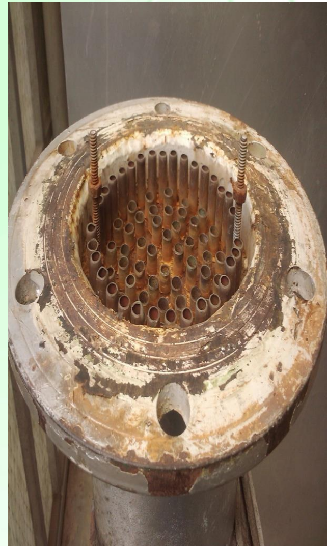
Liquid Redistribution unit in the new modified water scrubbing tower at IIT Delhi
